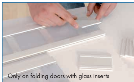
Only on folding doors with glass inserts Glue the end panels with double-sided tape at the bottom of the shortened plates
