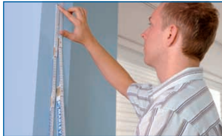
Measure the door opening (width and height)
