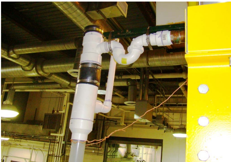
Figure 1 - P-trap (1-1/2 inch pipe size)
