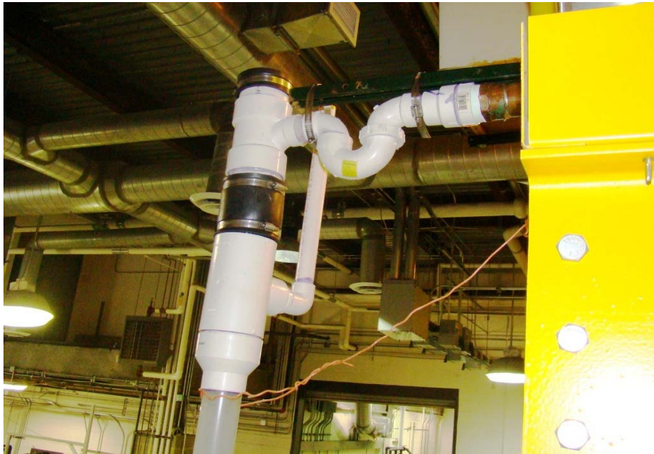
Figure 1 - P-trap (1-1/2 inch pipe size)
